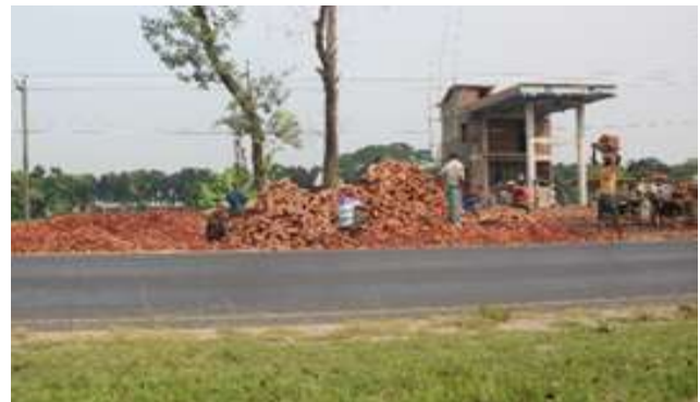
(c) Stack of construction materials.
