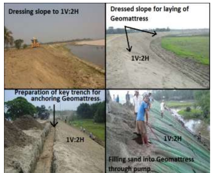
Fig. 5. Installation of Geotextile mattress at various stages
