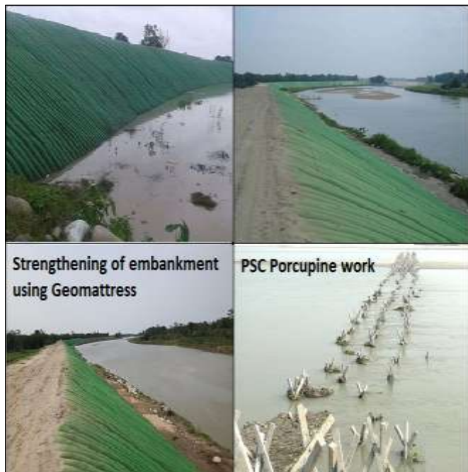
Fig. 7. Implementation of geotextile mattress and porcupine works
