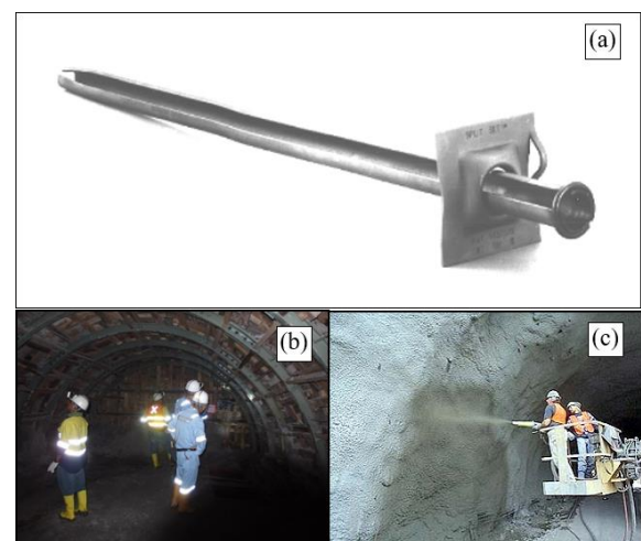
Fig. 11. Support systems for roof and sidewalls of mine tunnel (a) Friction rockbolt (b) Steel arch (c) shotcrete
