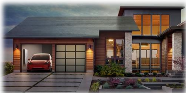
Figure 3: Solar tiles used on a residential building
