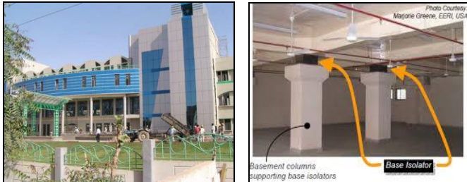
a. Bhuj Hospital Gujarat, India. b. Seismic Rubber Bearing.
