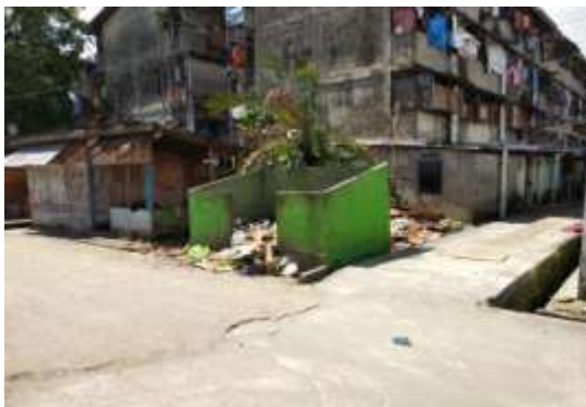
Fig. 2. Existing condition of waste collection in Sekanak
