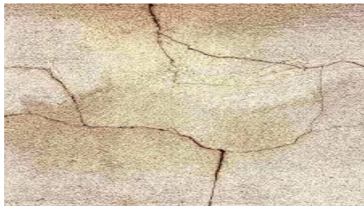
Fig. 3. (a) Thin crack (<1mm) (gharpedia.com)
