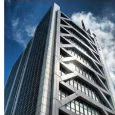
Fig2.6 Eccentric bracing
