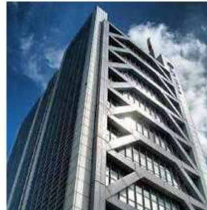
Fig2.6 Eccentric bracing
