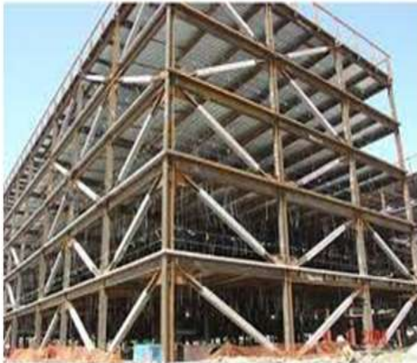
Fig 2.7 Buckling Restrained Brace
