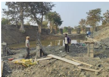
Fig.3. RCC columns newly constructed upstream to the KT weir for debris control.
