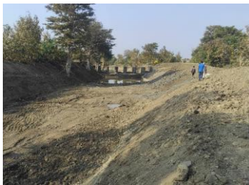
Fig.1. Upstream view of KT weir before construction of protective columns
