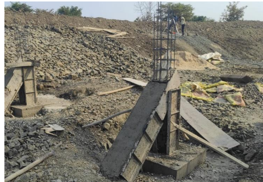
Fig.4. Side view of the RCC column arrangement
