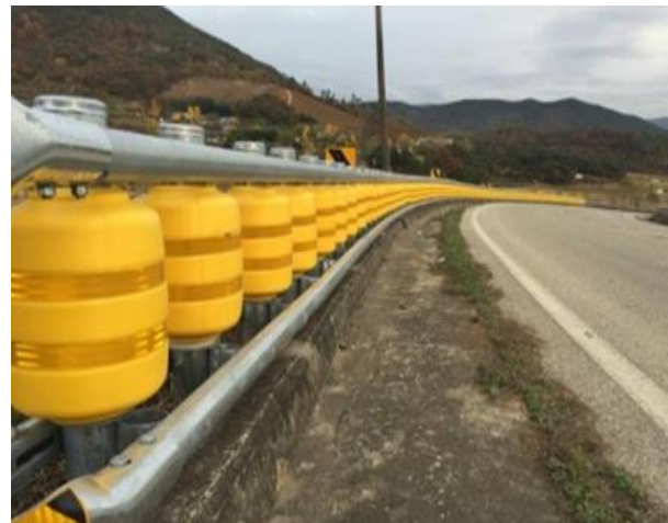
Fig. Rolling Barriers on horizontal curve
