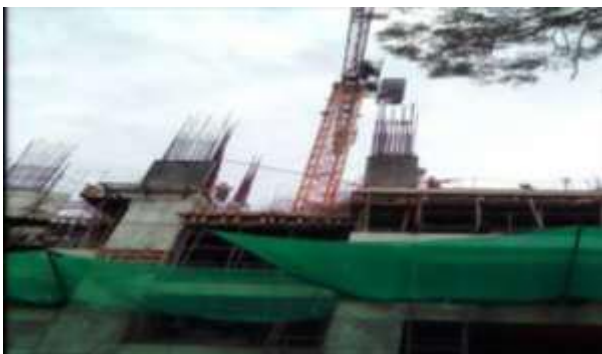
Figure.No.1 Mega Crane
