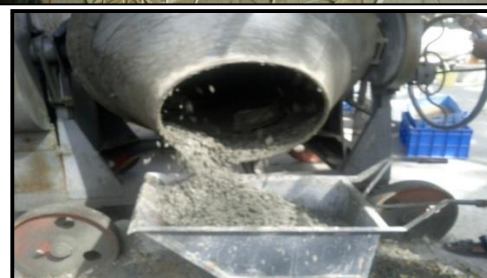
Fig.2 .Mixing Of Concrete
