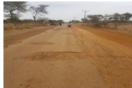
Fig. 3.2: Raveling (from visual site survey)
