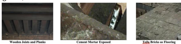
Fig. 4. Section of Flooring
