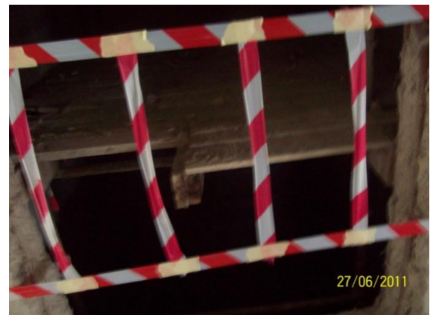
Fig 7 Warning Tape Showing there is an Open Hole
