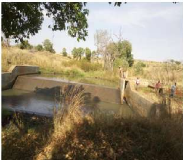
Figure 2.1: Diversion weir of Golda small scale irrigation scheme
