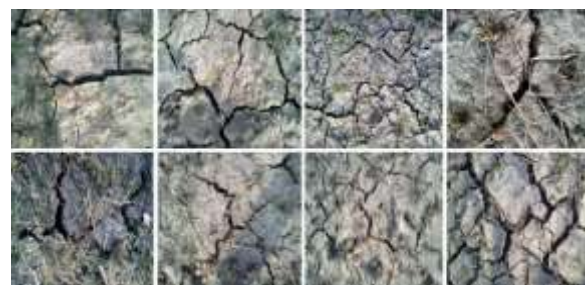
Fig.2. Cracking due to failure of clay soils
