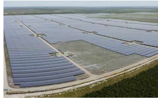
Figure3: Cestas photovoltaic park, connected to the network
