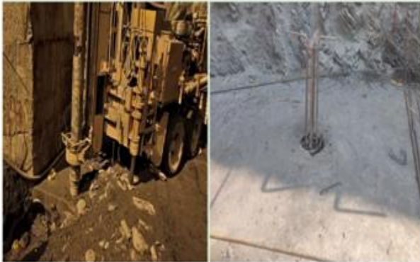
Fig. 5. Picture (a) Showing drilling equipment while drilling hole for micro-pile and Picture (b) Showing final micro-pile hole from top of the surface after complete reinforcement & concrete in Tehri PSP outlet foundation area.
