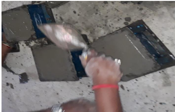
(b) Smoothing the top layer of mix
