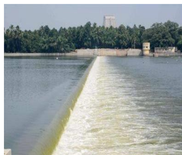
Fig. 2. Geethapuram shutter dam
