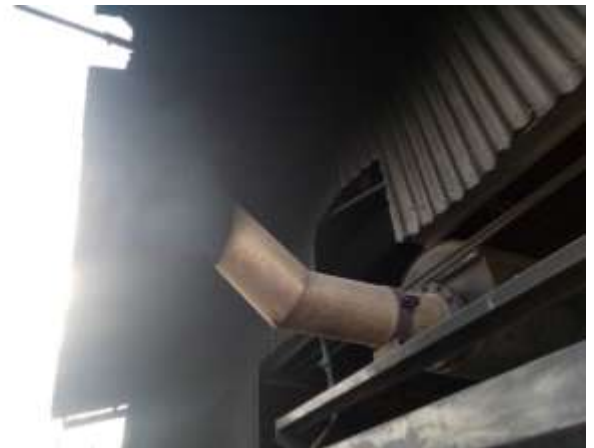
Fig. 30 Exhaust System of the Diesel Engine
