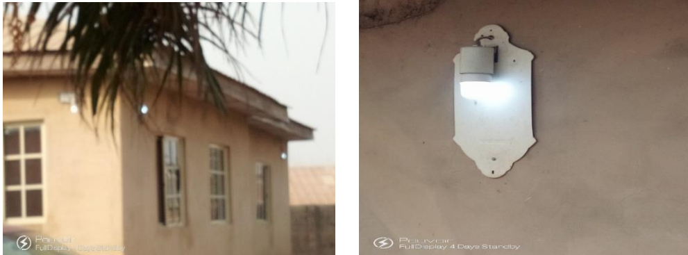
Fig 2: Power wastage through lighting during daylight
