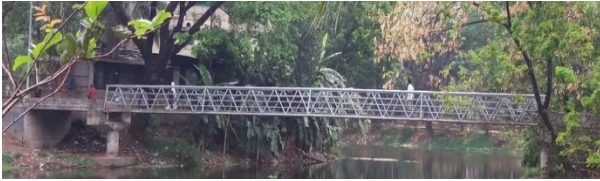
(a). Pedestrian Bridge
