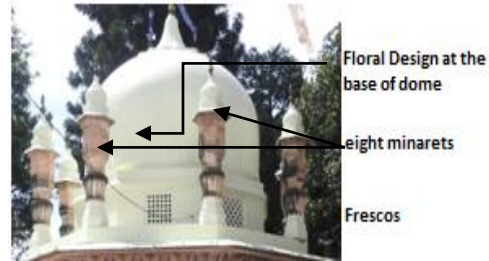
Fig.20 Dome at Samadhi
