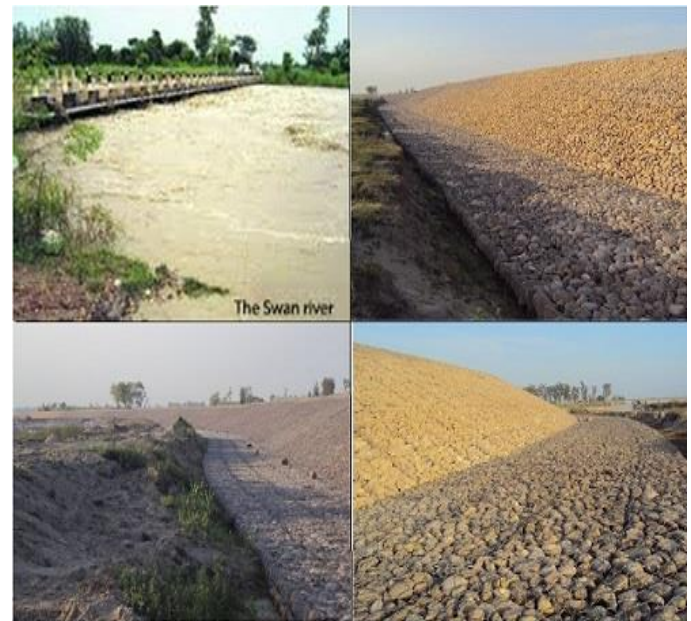
Fig. 4. Completed embankment in Phase-II
