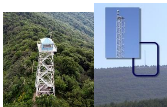
Fig.1: Platform for early forest fire detection fixed with towers and specialized cameras
