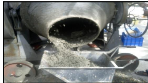
Fig.2 .Mixing Of Concrete
