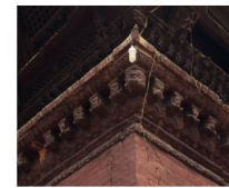
All layers of Cornice Exposed
