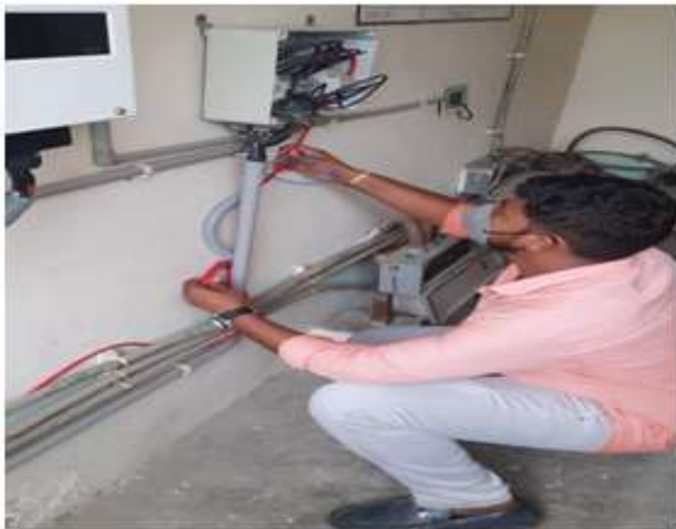
Figure 6: Technician providing dedicated DC Earthing
