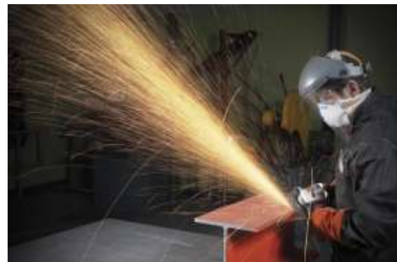
Figure 3: Disc grinding operation in steel beam (collected from Google images).
