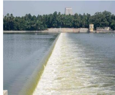
Fig. 2. Geethapuram shutter dam
